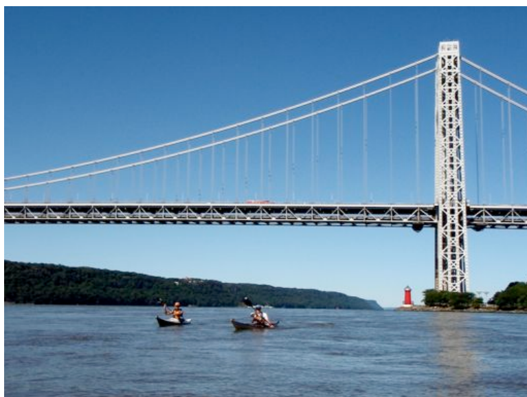
The massive George Washington Bridge, with its famous Little Red Lighthouse, was the last of our 21 bridges.
