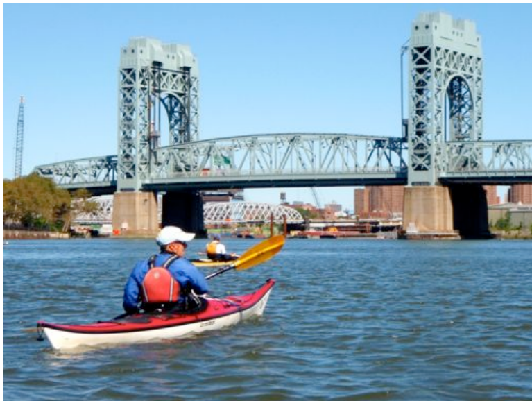
The Triborough Bridge is one of 12 along the 8-mile long Harlem River.
